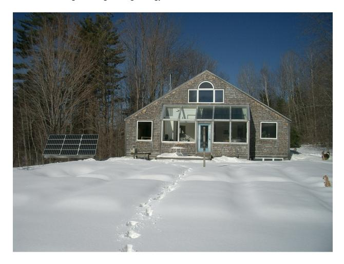
Integrated architectural and engineering design and construction for a private residence in Meriden, NH. This superinsulated home uses passive solar and wood-fired heat and hot water, and is designed for health, comfort, and durability. A ground-mounted utility-interactive photovoltaic array supplies about 60% of the annual electrical usage.
