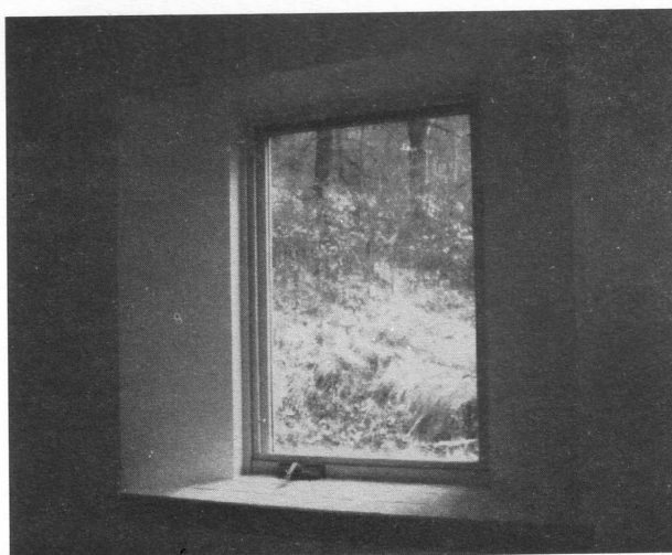
The deep window wells are splayed for better light distribution into the house. This casement window has an insulated fiberglass frame from Owens Corning and super-high-performance Heat Mirror® glazing from Southwall. Source: Marc Rosenbaum
